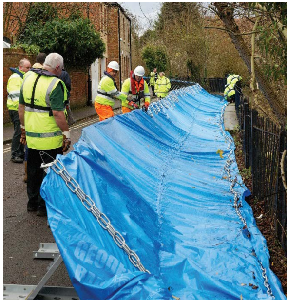
Temporary flood barriers being assembled
