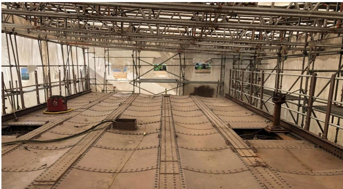
Now that the top of the bridge is complete, the blasters can return to do their final surface clean before the painters come to tidy up the undercoat and start the painting in earnest. Each of the elements has to be painted to create a safe surface to help prevent against future corrosion and, with so many different elements, including all those rivets, it will take four to five weeks to complete this work.
