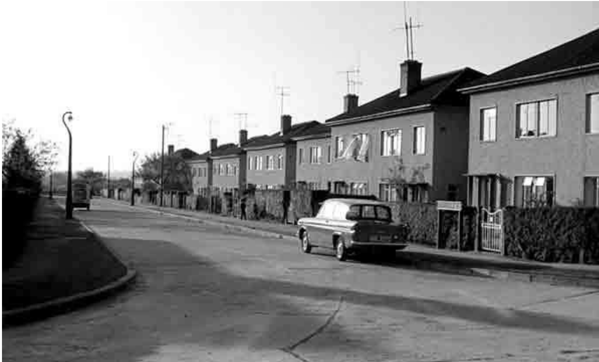
Orlit houses on Wynbush Road in 1967, having had their roofs raised and their concrete walls coated in pebbledash. Image from the Oxfordshire History Centre, POX0221822.
