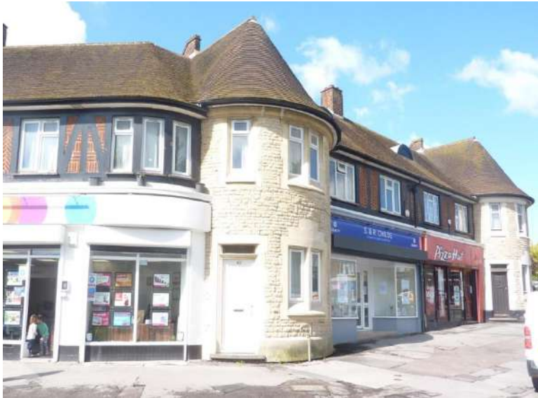
The parade buildings are thoughtfully designed, with deep roofs, stone-clad semi-circular turrets (giving access to the flats above the shops) and decorative half-timbering and brickwork panels.
