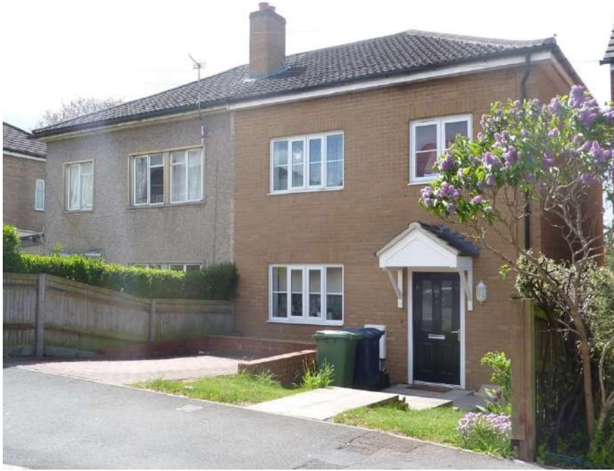
(Left) possibly the last remaining original Orlit house on the Rose Hill estate, on Nowell Road, and (right) its semi-detached pair which has been rebuilt in brick.
